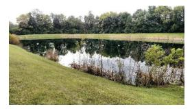
4. Pond II: This pond is located right off the street at Settler's Bay and is equipped with a fountain (aerator), as well as a dedicated electric utility box. The pond was without riprap, had some debris with moderate shoreline erosion.
