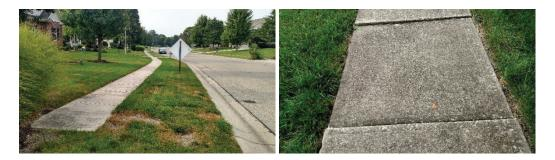
10. Sidewalk with School Access: This walk was segregated as it is uniquley situated and may have requirements for replacement. Some cracks were also noted here.
